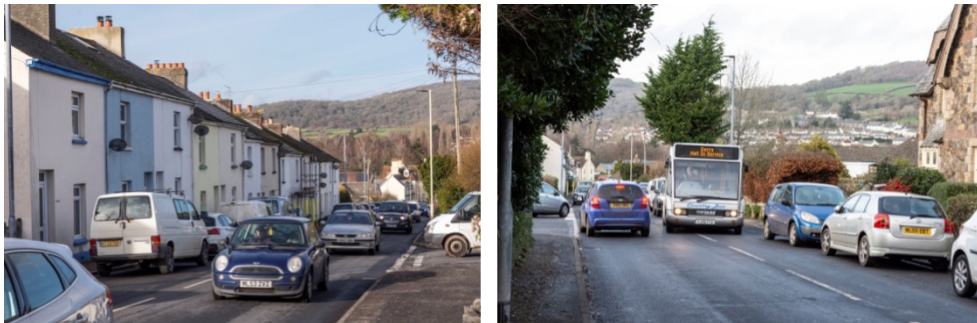
Fig 6.4 Roads adjacent to a mix of residential property off Newton Road
