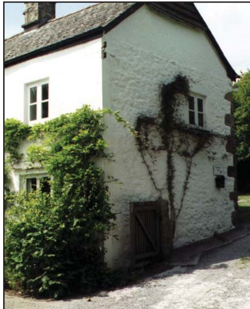
Figure 2 The gable end of Little Mead that was probably hipped or half-hipped when the roof was formerly clad in thatch.
