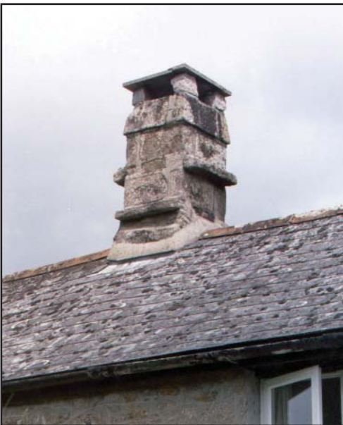
Figure 1 The weatherings inset into this stack suggest the roof was formerly clad with thatch.
