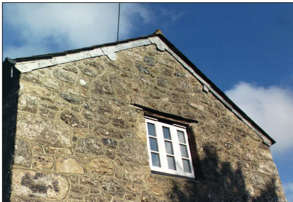
Figure 3 The use of slates to protect roof verges is a distinctive feature
